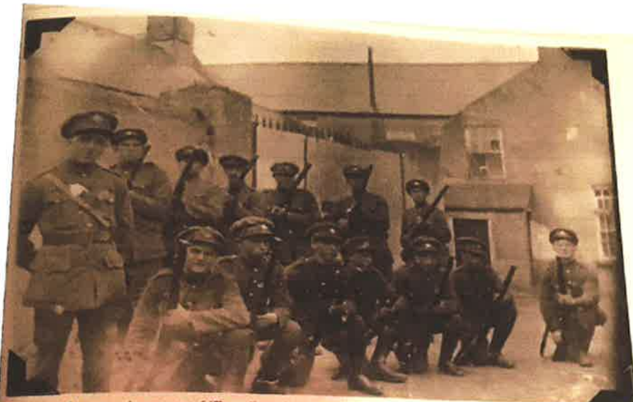
Present Arms – A group of 'Free State' soldiers in the yard of the RIC Barracks on Main Street in 1923. The 'Free Staters' moved in when the RIC and Tans evacuated the building after the truce. The building is now the Griffin Arms Hotel. Paddy O'Meara in Officers Uniform on the extreme left and Jack Kearney – St Brigids Avenue kneeling on the right of the photo. The identification of the rest of the group is not known. Photo: Rev. P. Cleary
